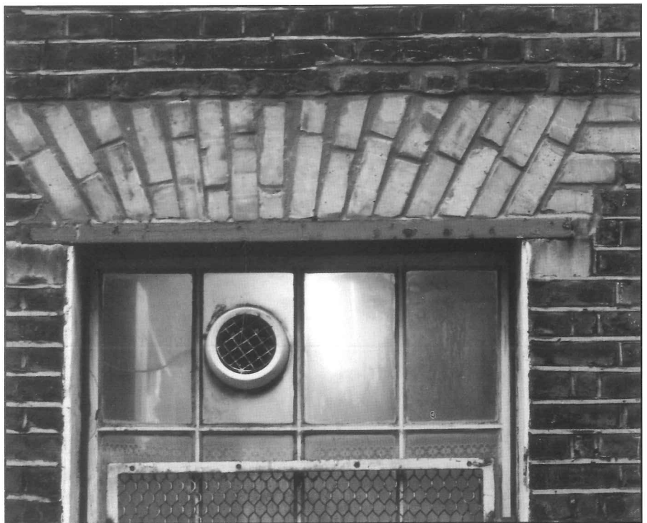
Crude replacement of a gauged window arch. Work of this low a standard deprives a building of its historical and architectural interest and lowers its value too.
