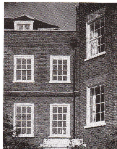
Windows are a useful guide to the dating of a house: here it can be clearly seen that the bay on the right has been added to an earlier house. The window with horns is an even later replacement
