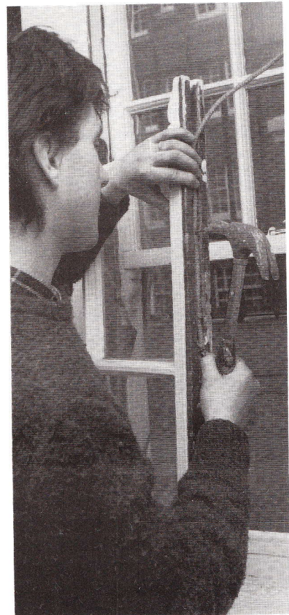
Fixing new cord to sash
