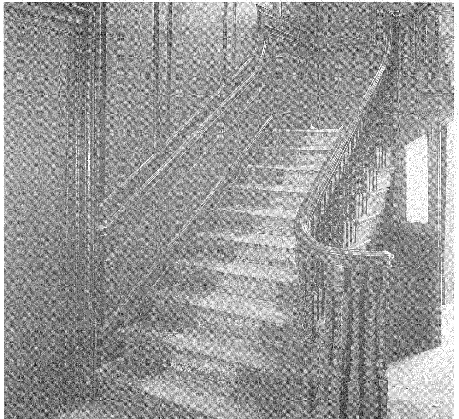
Fine raised and fielded panelling in an early eighteenth-century house at 4 Fournier Street, Spitalfields
