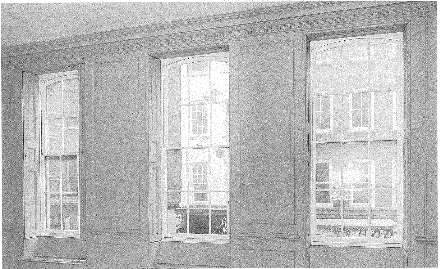
67 Dean Street, Soho, c 1732; the first floor room has built in window seats, recently restored
