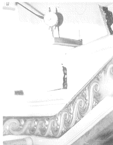
A dial gauge being used to read deflection of the stair during a carefully-monitored 24-hour load test
