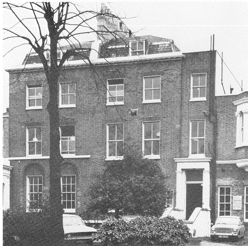
A pair of semi-detached houses with mansard roofs and hipped ends finished with lead rolls
