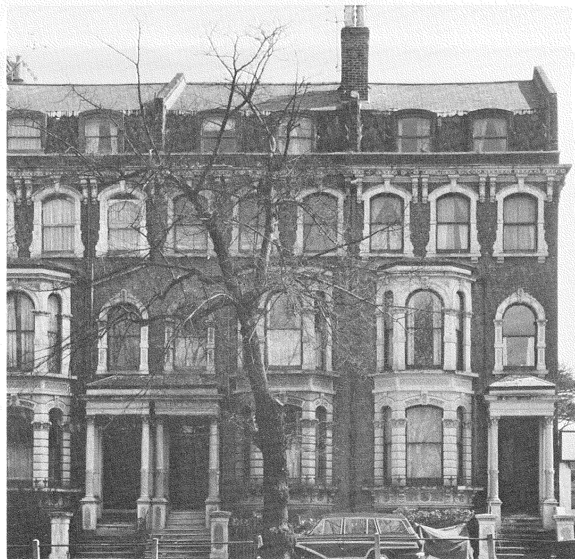
A Victorian terrace with three windows on the second floor of each house and two dormers above. The shaped slates of the lower slope and the curved tops to the dormers are appropriate features for this particular terrace but would not be right in many other contexts
