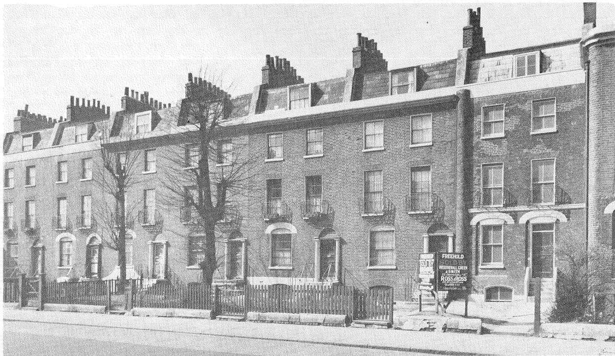
A terrace of London houses of the Regency period, showing mansard roofs with the party walls which follow the pitches of the roofs; the dormer windows are set behind the parapets and each two-bay house has one dormer
