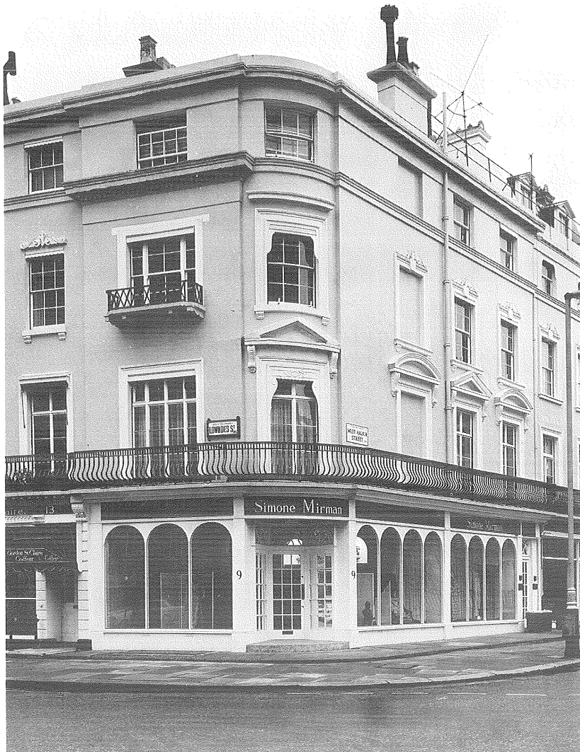
An example of a sympathetically designed twentieth-century shop front which replaced unsuitable plate glass windows
