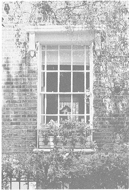
Wooden sash of the mid 1830s with decorative margin lights
