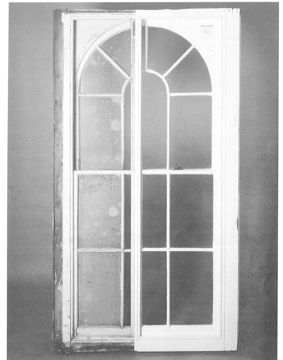
A late Georgian sash window of c1800, partly restored, from Greenwich, London
