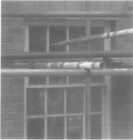
Opening the window would have avoided smashing old glass
