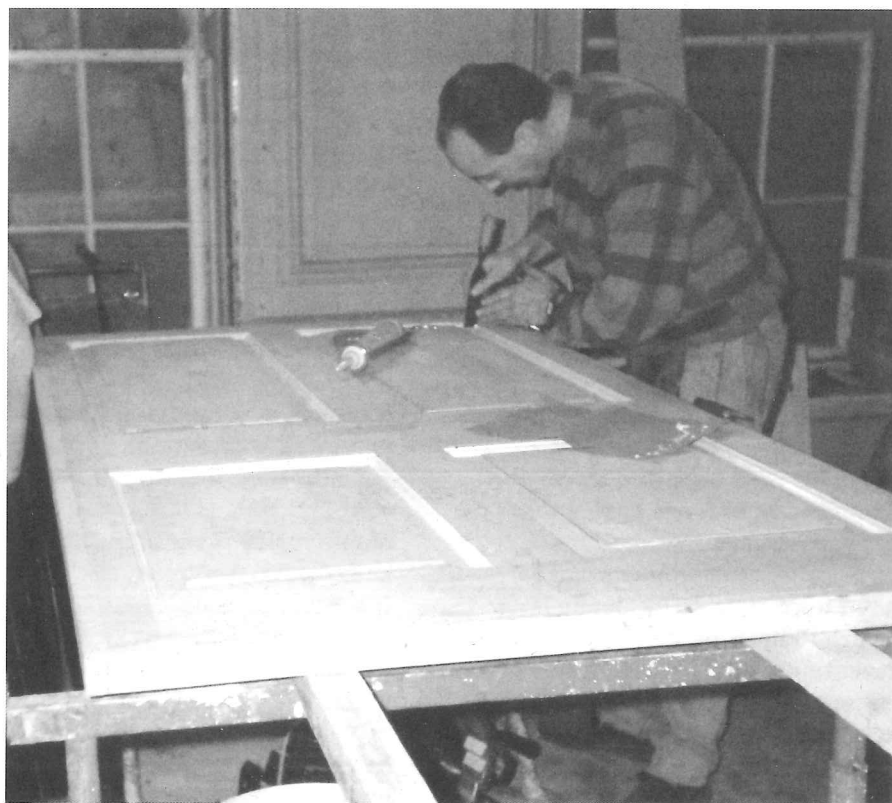
Intumescent mastic being applied to edges of upgraded door panels
